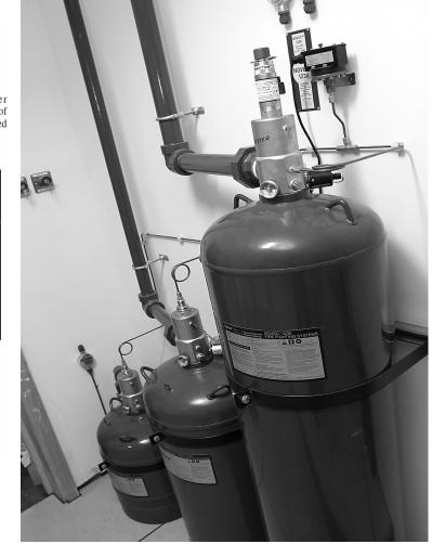
Existing halon 1301 pipework may be able to be re-used with Novec 1230 Fluid in some cases
