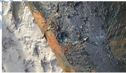
Pin hole in jet fuel pipeline.
