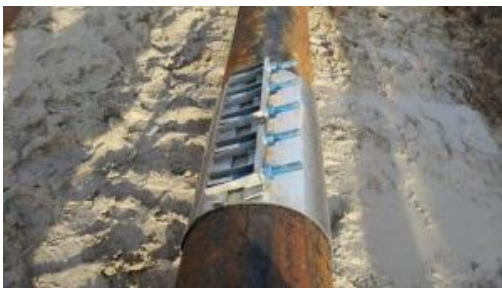
Repair to jet fuel pipeline.
