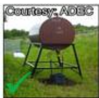
The tank legs or stand are in good condition and are on a stable foundation.
