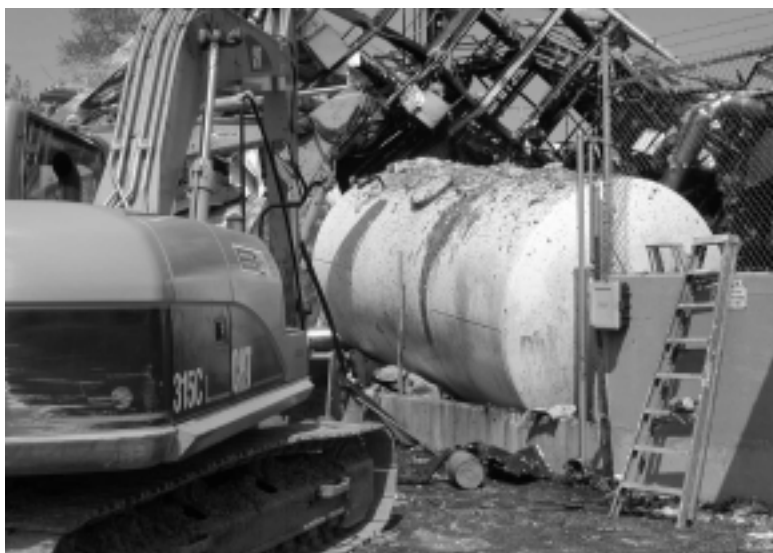
Figure 3. Aqua ammonia storage tank prior to removal from diked area.
