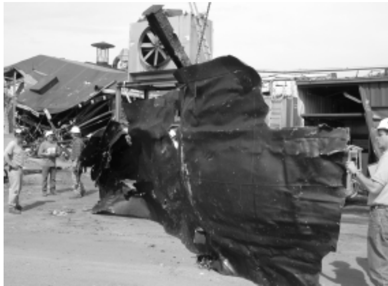
Figure 6. Feed tank #2 shell, after recovery.
