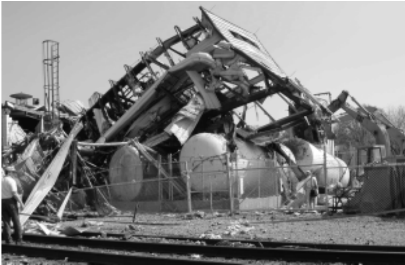
Figure 11. Collapsed spray dryer structure.
