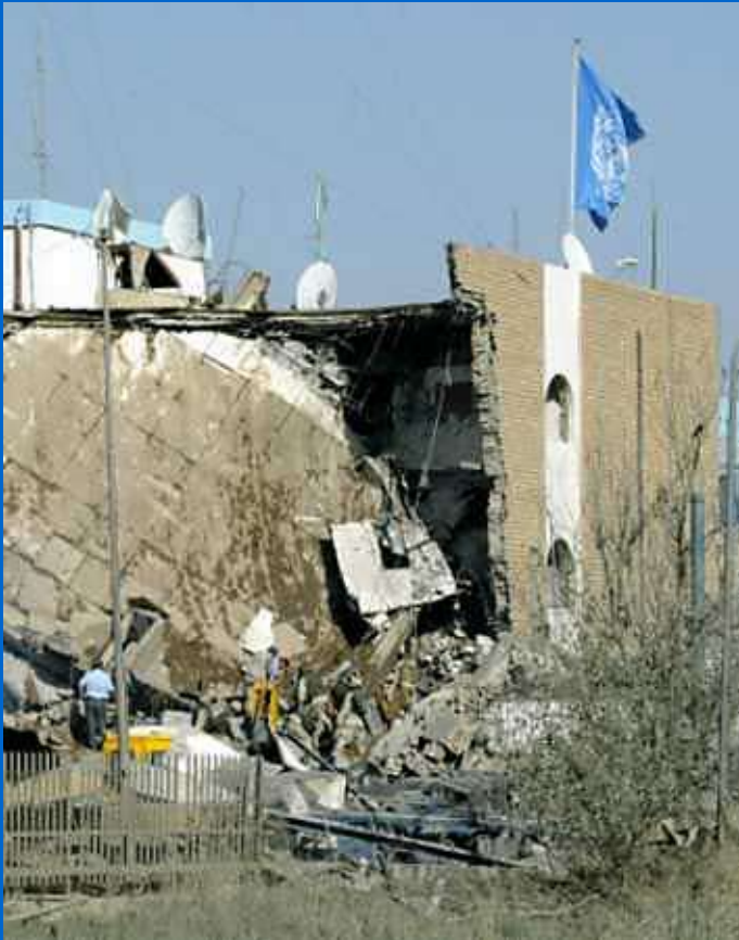
U.N. Compound Blast – Iraq: 19 Aug 2003
