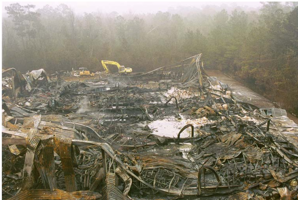
Figure 7. Remains of ACS warehouse viewed from compounding area.
