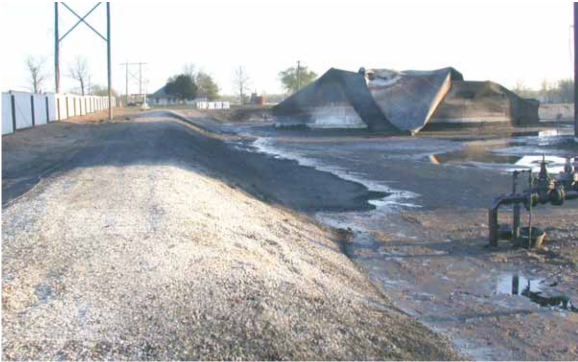
Figure 2. View of wreckage of tank 11 facing south. Note power lines and earthen dike at left and overpressure piping at right.
