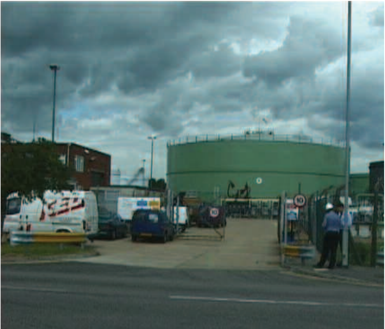
Figure 2 Looking into part of the Buncefield site before the incident. Note the ground vehicles, large storage tanks, and occupied buildings. To the right are manifolds that distributed fuel around the site
