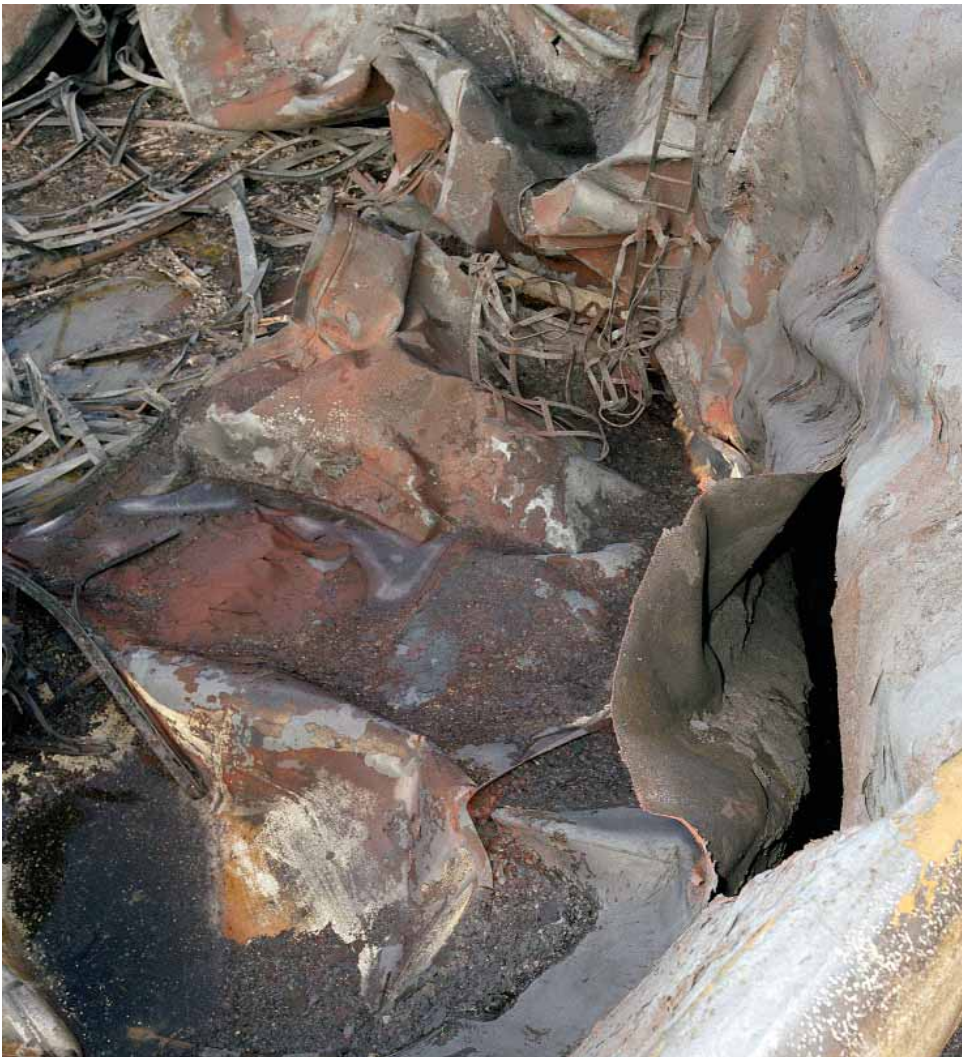
Figure 9 View into Tank 912
