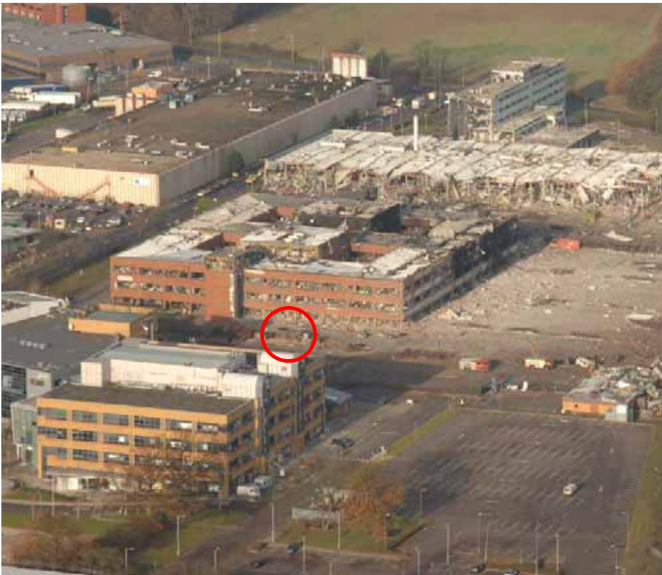
Figure 12 View looking north towards the Northgate and Fuji buildings, with the Buncefield depot just off picture on the right. The emergency generator cabin is highlighted
