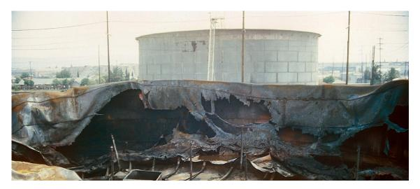
This keeping the wall from folding in <u>was</u> very important when the foam being used in Protein based because Protein based foams do not easily spread through one of these tunnels. If a AFFF type foam is to be used it is not as important to hold up the tank wall because the AFFF foams are very fluid and they spread through the tunnels much easier. Protein based foams are much more rigid that AFFF foams.
