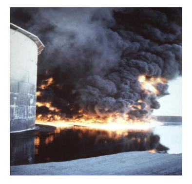
1. Very quickly cool other tanks that have <u>direct flame impingement</u> to there tank walls!
