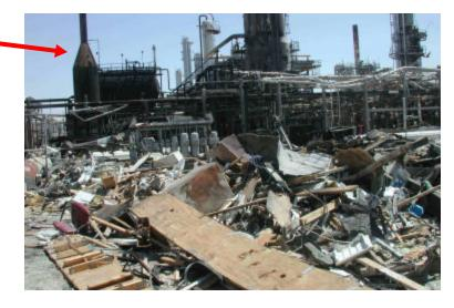
Some of the other trailer offices just feet away were damaged by the over pressure waves braking in the windows and doors in then pushing up on the roof, but these were **not totally destroyed** like the ones where the vapors got underneath them before the ignition The wreckage on the ground in the picture, came from the adjacent trailers that were destroyed. See below.
