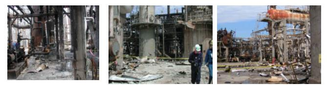
This is not the only time that major blast damage and resulting overpressure damage has occurred <u>at the edge of a vapor cloud</u> where the vapors were trapped under a structure.
