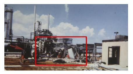
The Hydrocarbon processing industry should step-up their assessments regarding pressurization of structures inside and around process units. The industry has pressurized occupied buildings because of the electrical classification and personal protection, but not to prevent these buildings for becoming epic centers of explosive overpressures.
