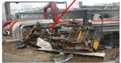
Below is what is left of a small motor control center (was in the red box) after a propane vapor cloud covered this area with enough depth to get in the MCC through the air conditioning air inlet. The floor of the MCC was all that is left in place after the racks were moved out during the investigation. Note the control room on the right, no vapors entered the building because the air intake was on the roof, even though it was much deeper in the vapor cloud.
