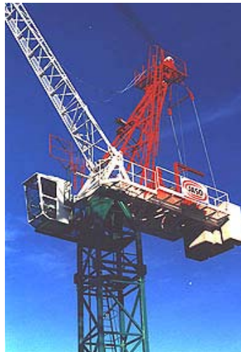
Photograph 1: Luffing jib tower crane similar to that involved in the accident
