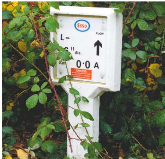
Oil pipeline marker post.
