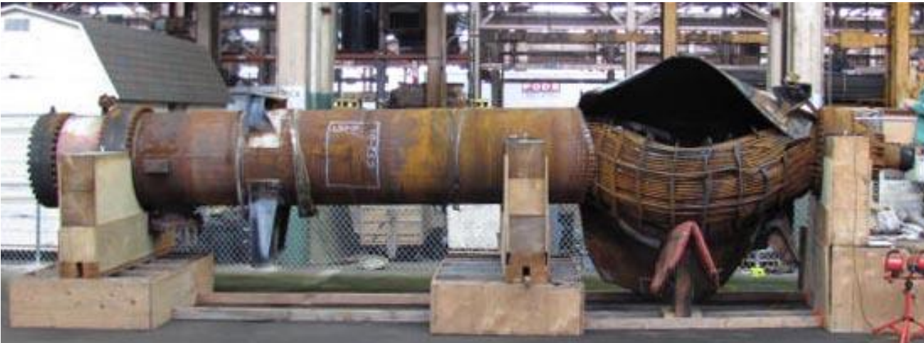
Photo 1: Sections 1-3 [from left] showing failure locations
