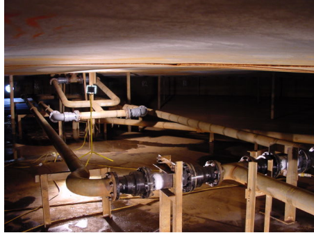
Figure 2 – Articulated Roof Drain System
