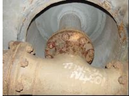
Figure 3 – Roof to Drain Connection (prior to failure)
