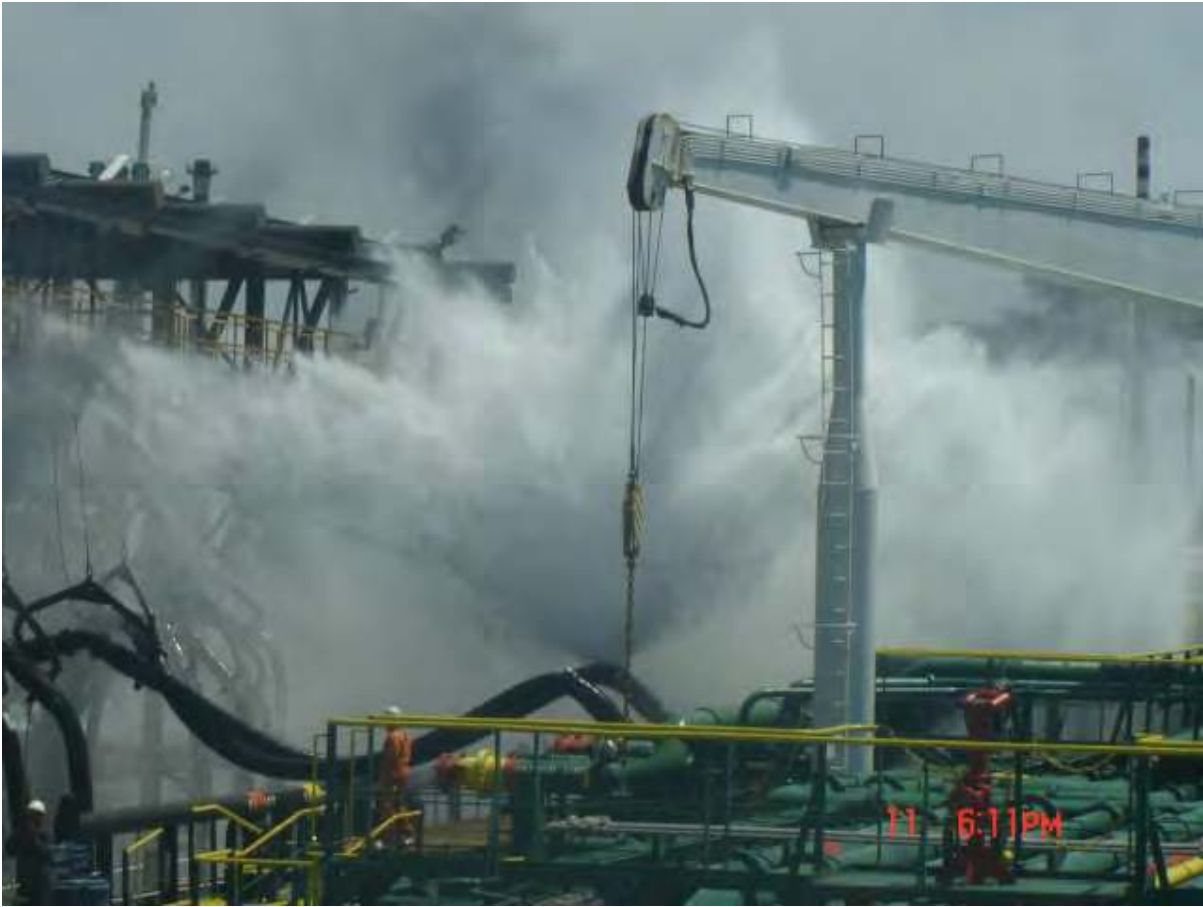
ograph 1 Leak from hose prior to fire.
