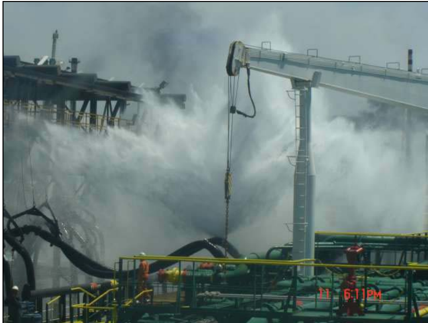
Photograph 1 :Burst of cargo hose before fire.
