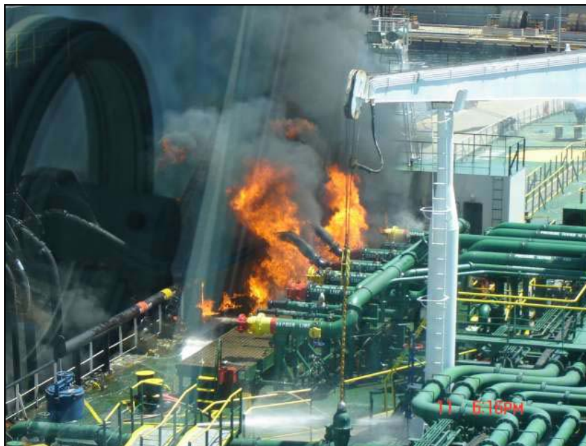
Fire burning on jetty and vessel
