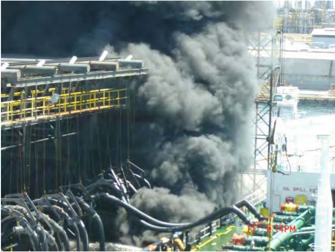
Fire burning on jetty. Note vessel's fire stream directed upon jetty in bottom of photograph
