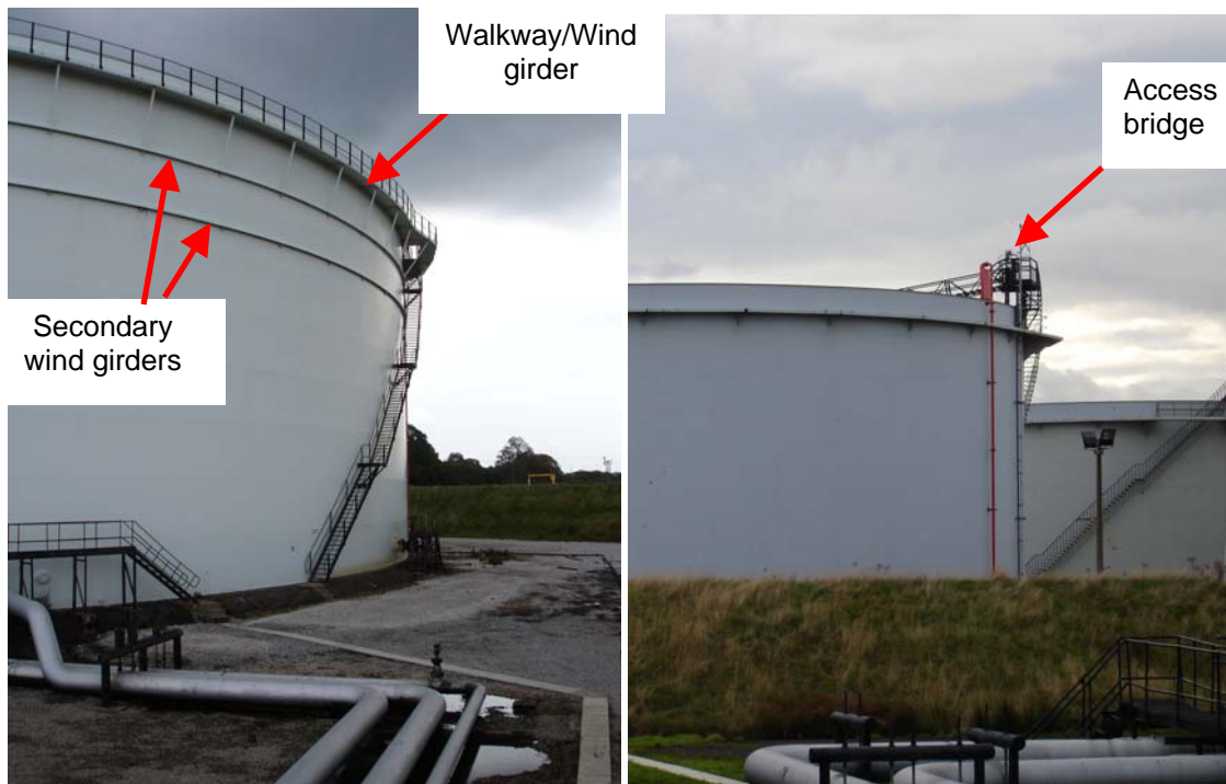
a.) FD tank with 3 wind girders
