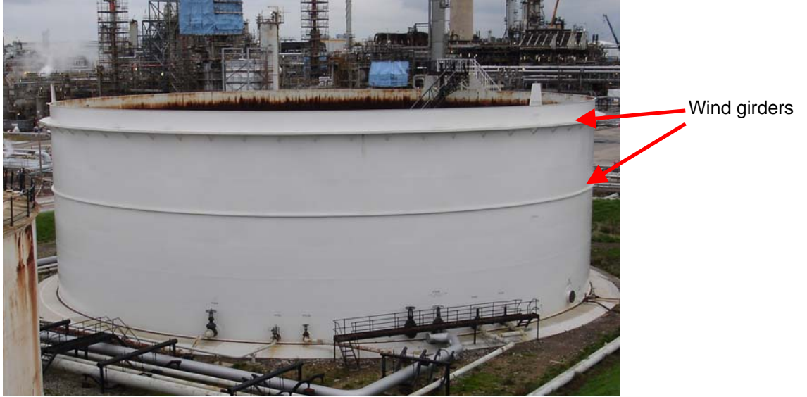
Figure 8c Another FD tank with different wind-girder design.
