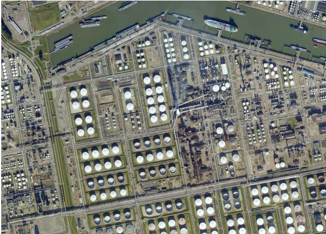
Figure 4 Example of part of a site seen from the air. Equipment characteristics of all the sites in the incident population need to be calculated – a major task.
