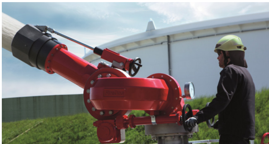
Fig. 3 Fire monitor in a test run at a tank farm
