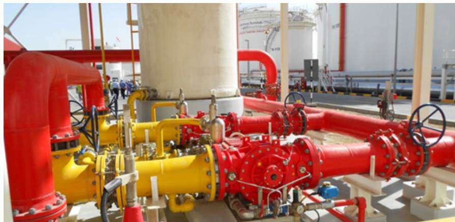
Fig. 4 Water motor with proportioning pump
