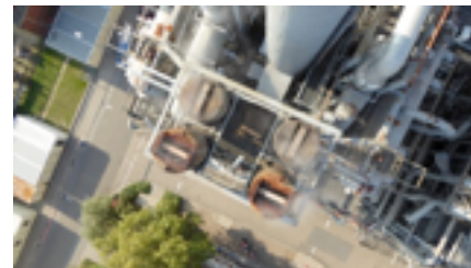
Inspection of silencer outlets
